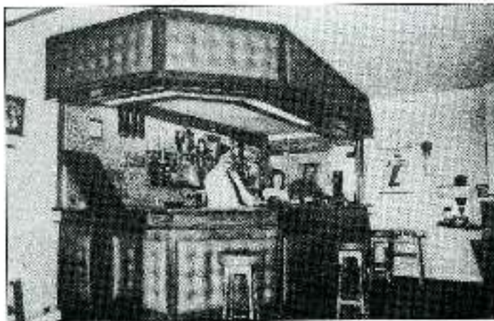
Clubhouse and bar renovations complete (1985)
